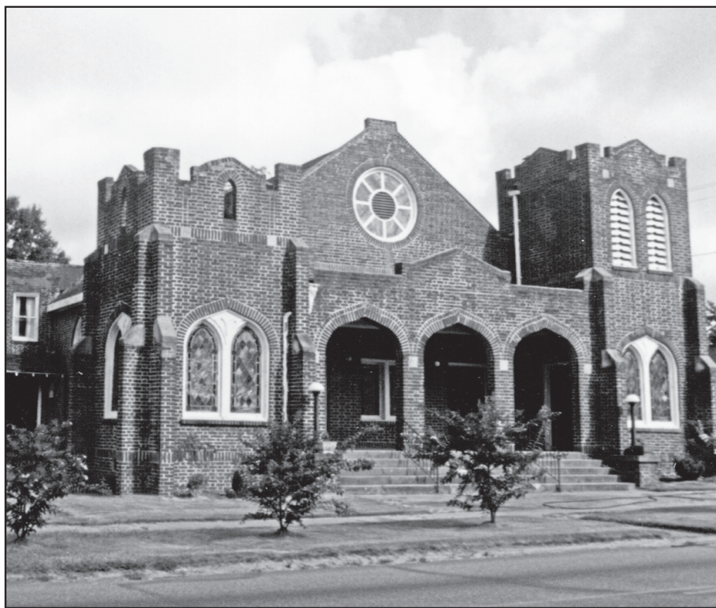
Sanctuary facing 2nd Avenue
